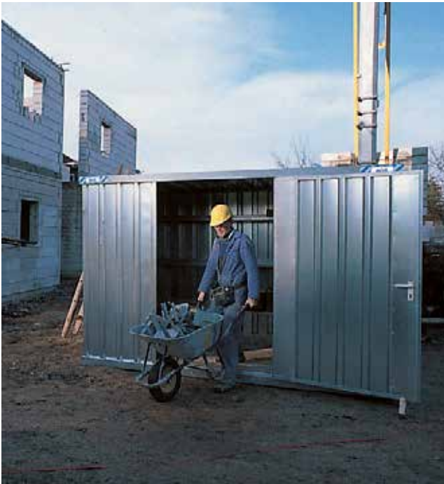
Building Site Container
