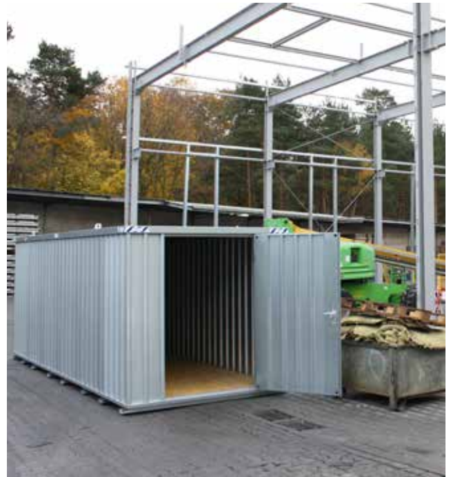
Building Site Container
