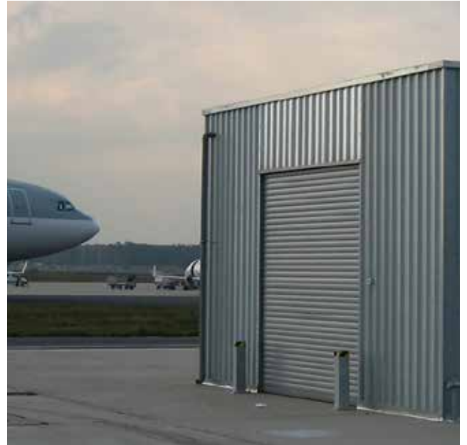
Material storage on the airport landing field
